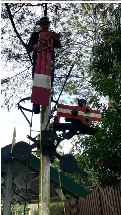
Warwick dismantling the old steel post fittings.
